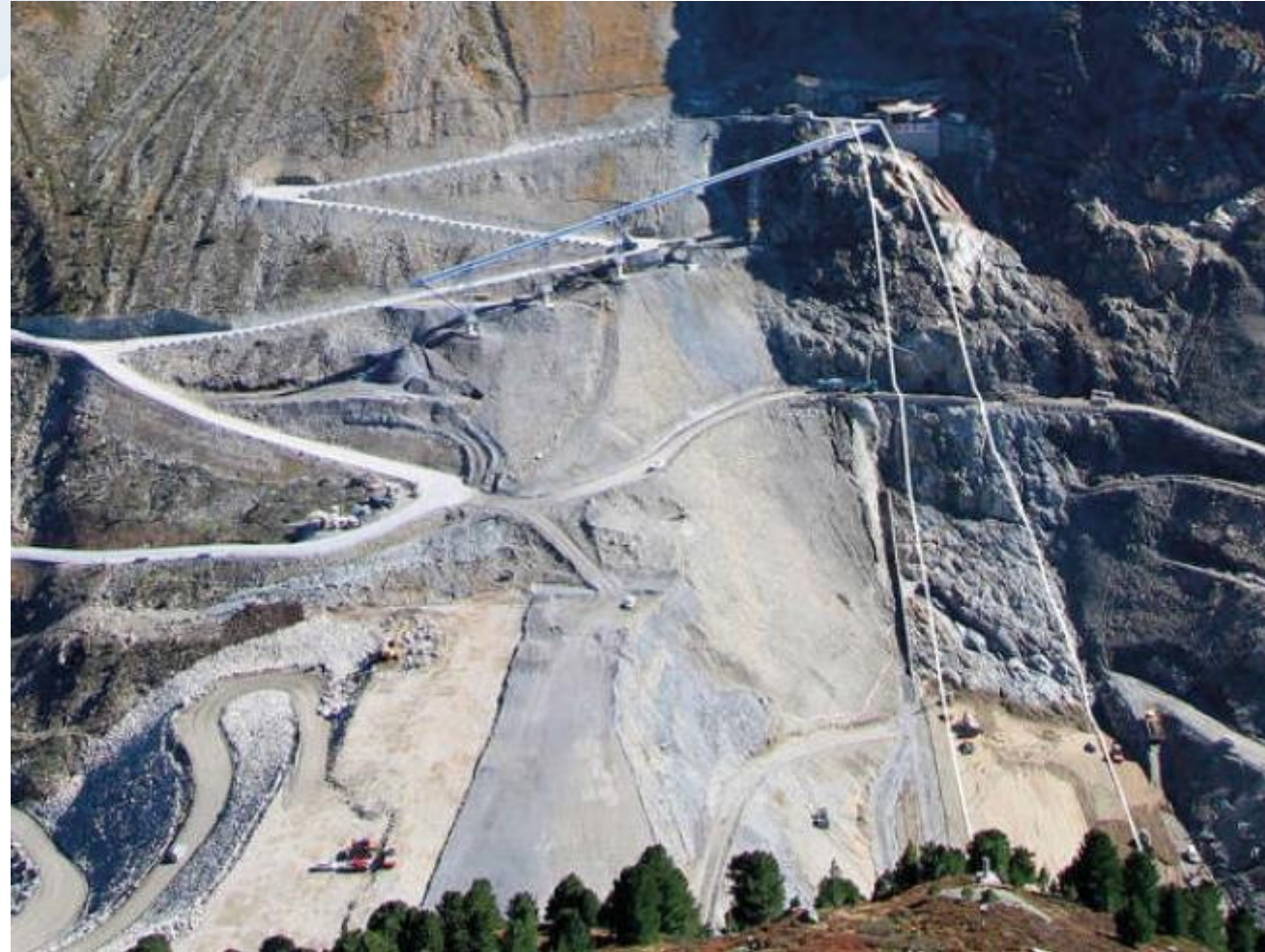
Construction of Kühtai PSH (2023) © Perzlmaier
