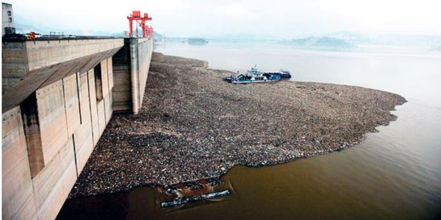
Fig. 1. Accumulation of floating debris behind the Three Gorges (Sânxiá) HPP dam on the Yangtze River, China [4].
